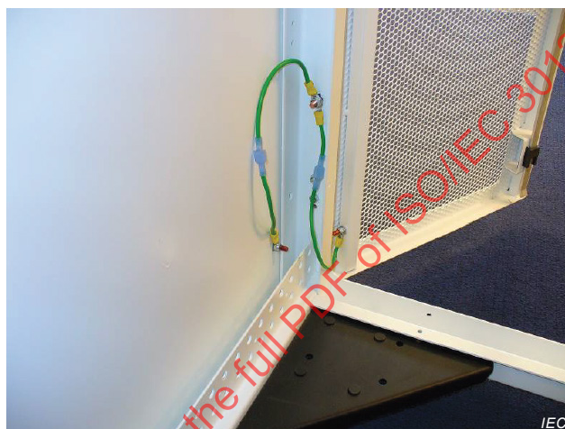
Figure 4 – Example of a bond connection from a cabinet to the cabinet door
